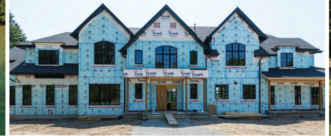
Exterior code board insulation is installed before the siding, adding further value to the home.
