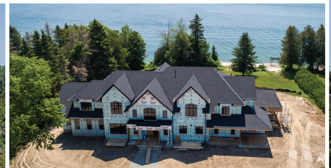
Exterior code board insulation is installed before the siding, adding further value to the home.
